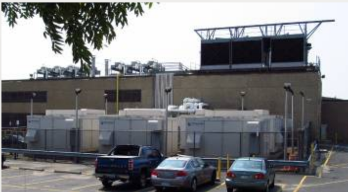
Fuel cell-based microgrid in Garden City, NY after Hurricane Sandy
